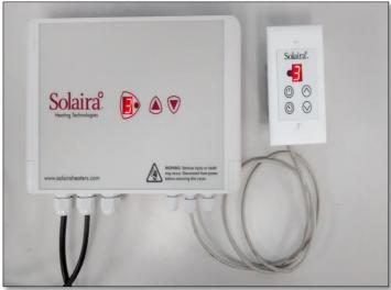
Switch SW2 on the main controller PCB should be set to "REMOTE COMMS" as shown in the picture above. When "REMOTE COMMS" is selected the front panel buttons and the infrared interface on the main controller is disabled and the unit can only be controlled from the wall mounted remote control unit.
